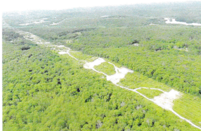
The new packed gravel access roads and pads on a right-of-way. Photo: CBS.
