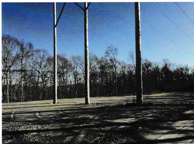
A large gravel-paved maintenance pad. Photo: CBS
